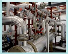
In the prototype, heat exchangers are 3 or 4 meters long. On a real scale, they reach a 12 meter length and a 4 meters diameter.
